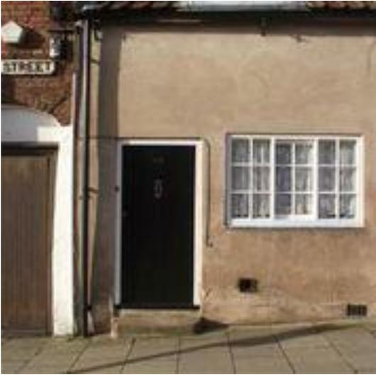
Plate 1: The front door and one of the horizontal sliding sash windows. The blocked off false door of the adjoining One-Stop shop can be clearly seen, viewed looking north-west.
