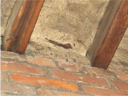
Plate 5: The beams, reed and plaster overlay in the ceiling of the passage between 63 & 65, viewed looking south-east.
