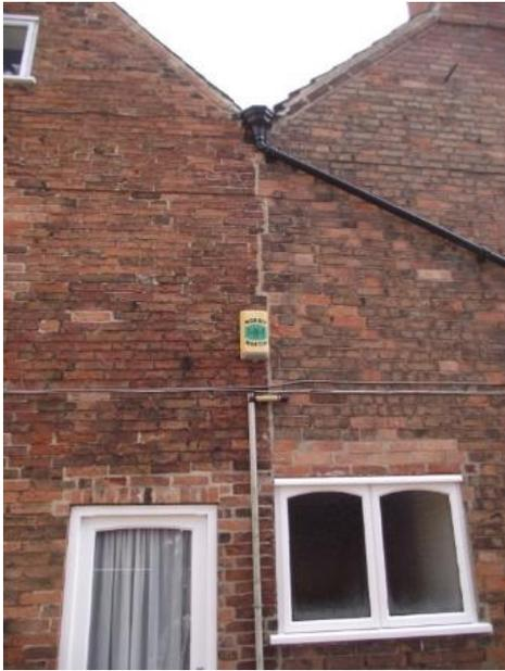
Plate 5: Building line between the two phases on the south-west gable, viewed looking north-east
