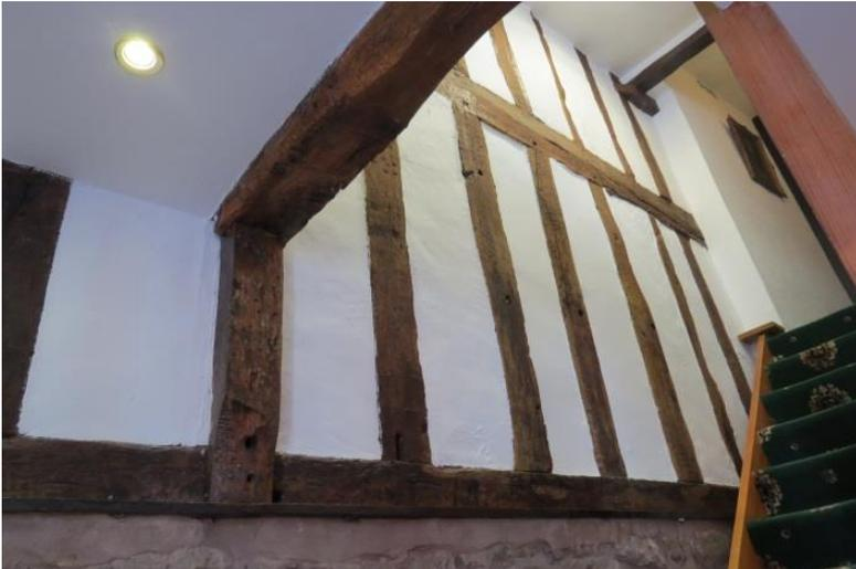
Plate 7: Interior view of timber frame and studding of number 64 viewed looking north-east in 62's entrance hall.
