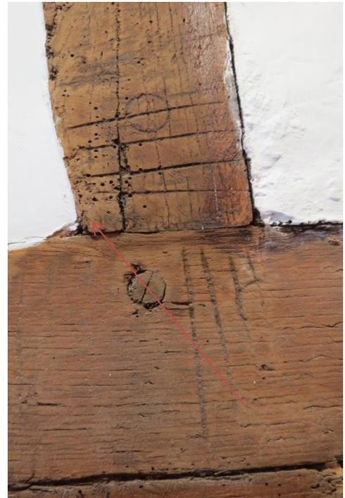
Plate 8: Carpenter's mark on joint 4 showing the 4 straight lines and a circle, viewed looking east.
