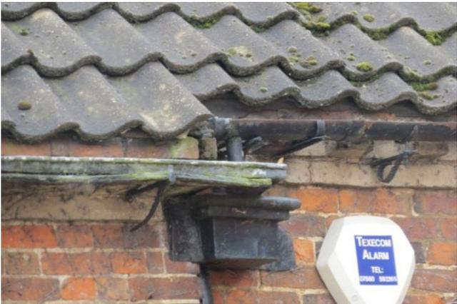
Plate 8: The header bricks supporting the gutter where phase 1 joins phase 2, viewed looking south.
