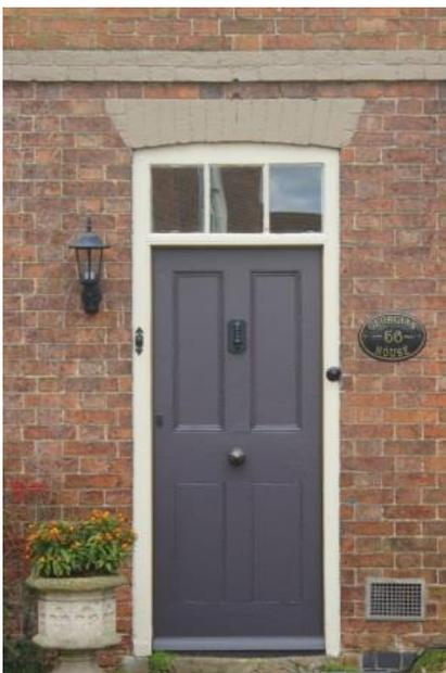
Plate 3: The central front door, cambered arch of rubbed brick and painted header brick, viewed looking south.
