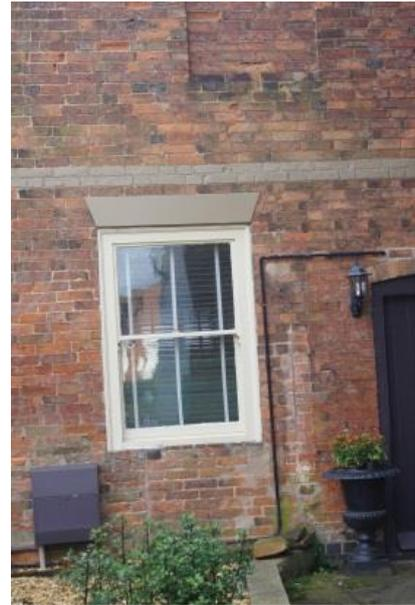
Plate 7: The lower front window and door in the cottage showing the altered brick work and false plat band viewed looking south.
