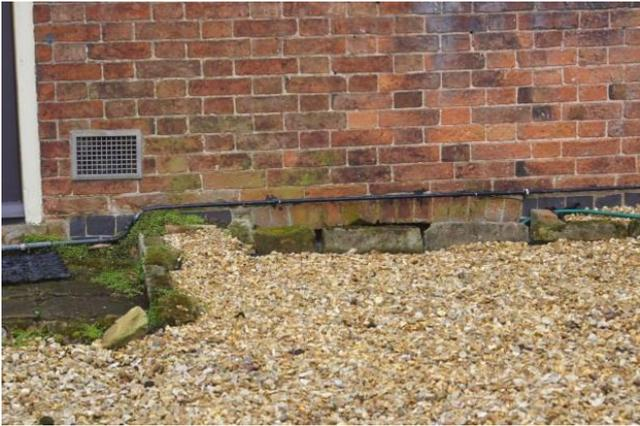
Plate 6: The curved brick lintel over the cellar window, viewed looking south.
