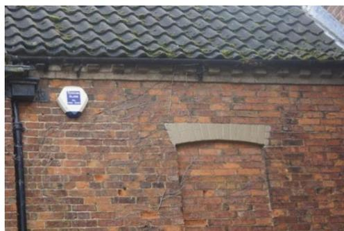
Plate 4: The bricked up single window and brick line under the gutter cornice, viewed looking south.
