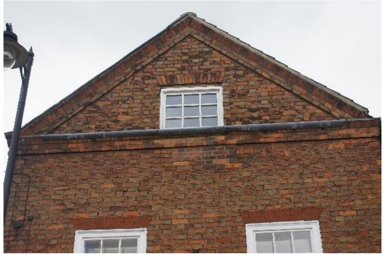
Plate2: Shop frontage showing eaves level string course, pediment cornice and rubbed and gauged brick flat arches , viewed looking south.
