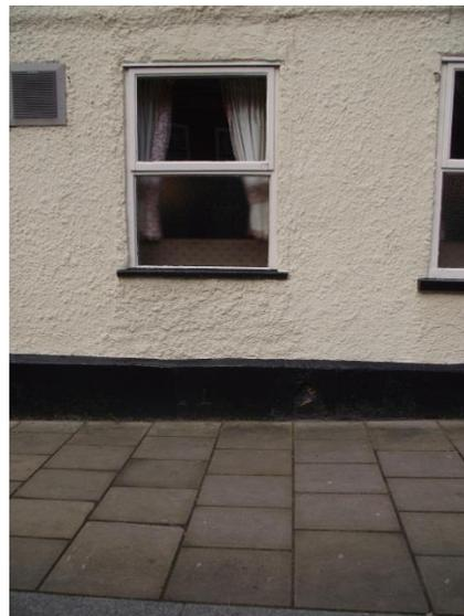
Plate 4: The boot scrapper in the plinth shows where the front door used to be, now a window, viewed looking west.
