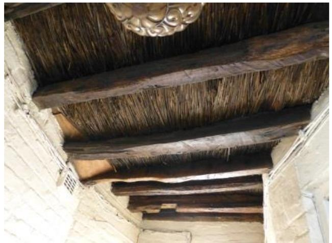
Plate 7: The beams and reed ceiling in the passage way, viewed looking south.
