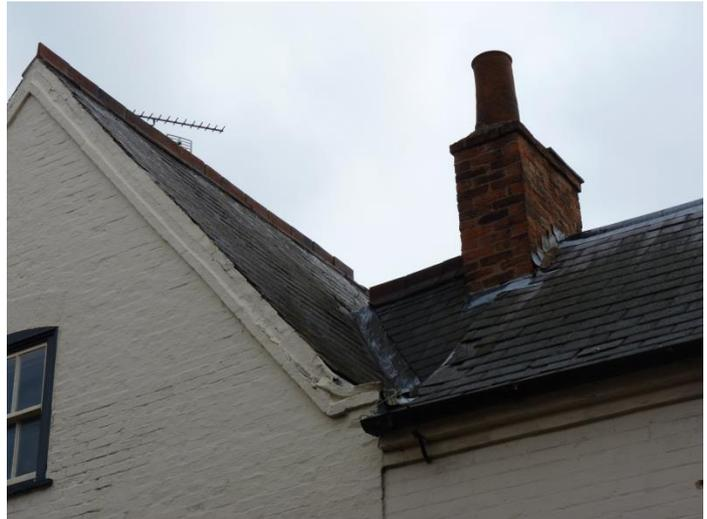
Plate 2: Plain dentilated header bricks on the front gable, viewed looking east.
