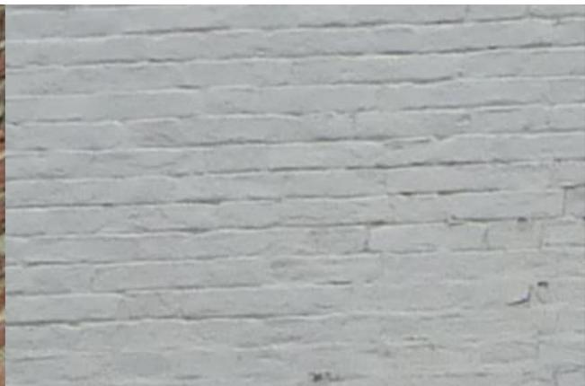
Plate 5: The bare, random courses of old 2 inch wide bricks many badly worn on the rear wall (a) compared to the colour washed front brickwork in Flemish bond with a few random courses.
