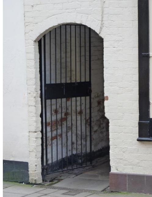
Plate 2: Gated passage leading to the rear topped with a rough brick segmental arch with tapered mortar joints, viewed looking south-east.
