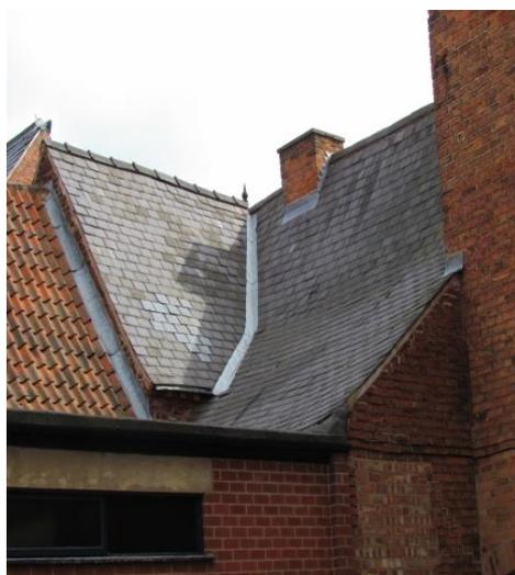
Plate 5: The rear roof of the front unit showing the out-shut (cat-slide) slope, viewed looking south-east.
