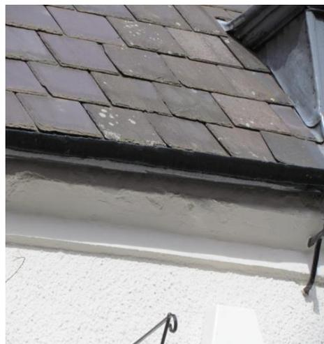
Plate 2: The slate tiles, lead flashing of the dormer and wooden wall plate, viewed looking north.
