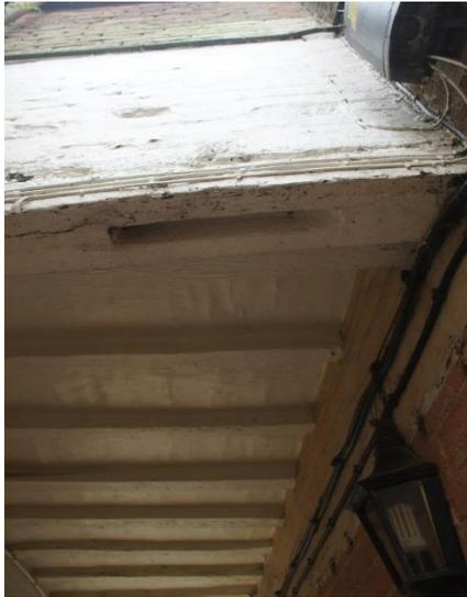
Plate 1: the passage way ceiling showing beams and mortice, viewed looking north-west.
