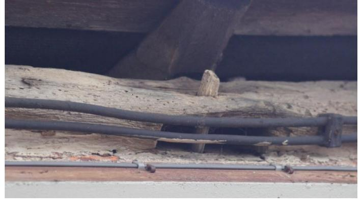
Plate 4: Detail of smaller mortice to house close studding in wall plate on north facing wall showing peg in situ, viewed from beneath looking south west.
