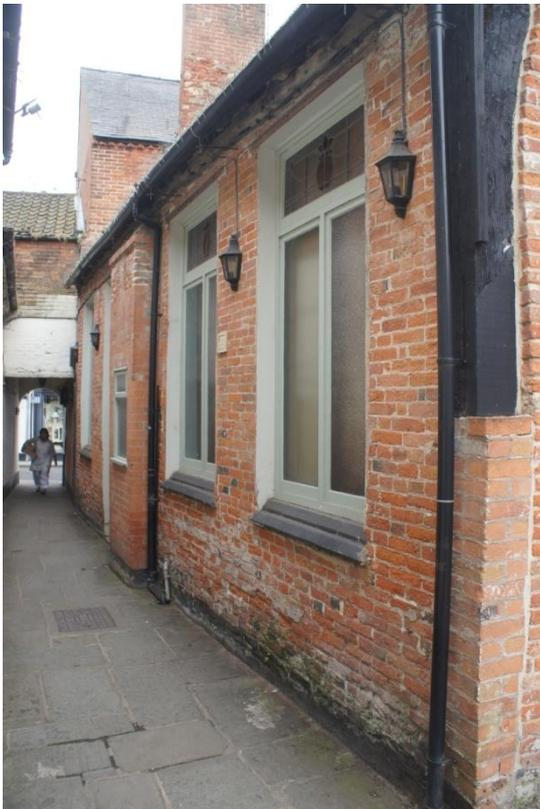
Plate 5: General view of NE facing brick façade supporting wall plate with mortices for close studding, showing brick columns replacing original wall post, viewed looking south-east.
