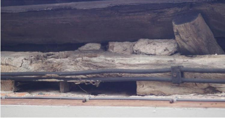
Plate 3: Detail of substantial mortice to house large wall stud in wall plate on north facing wall showing peg in situ and common rafter, viewed from beneath looking south west.
