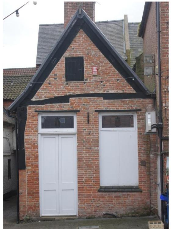
Plate 2: West facing gable end showing truss, brick infill, viewed looking south-east.
