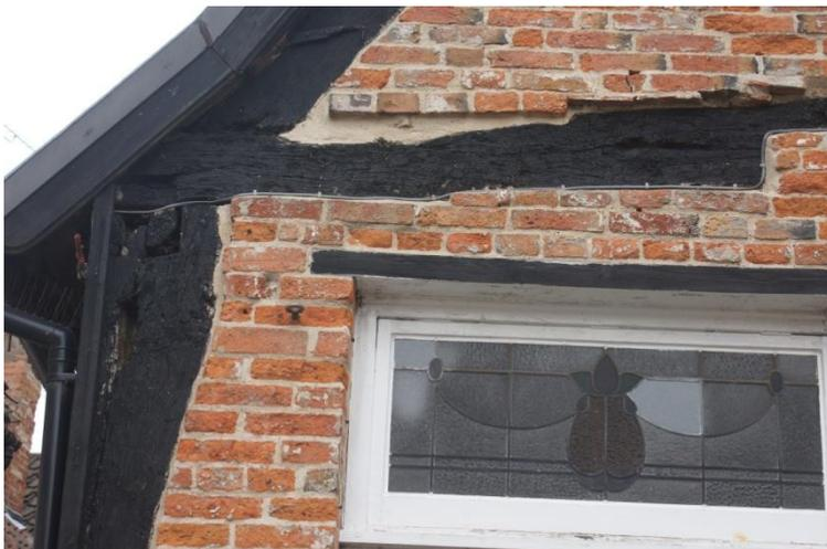
Plate 1: Detail of NW corner wall post joint showing jowled head with wall plate, tie and principal rafter, viewed looking south east.
