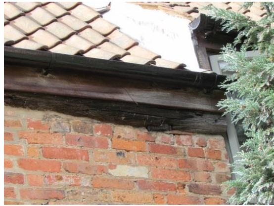
Plate 5: Wall plate and stub of vertical framing of no. 64a, to the left of the conifer in plate 4, viewed looking west.
