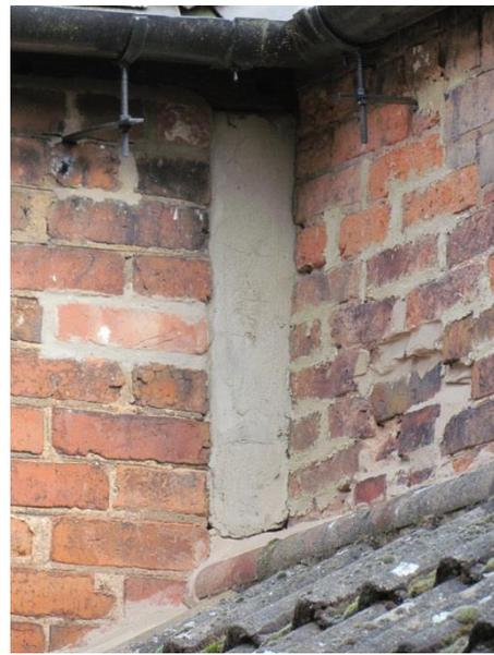
Plate 7: Render strip adjoining rear of nos. 64 and 66's rear extension, wall plate just visible at top, viewed looking north-east.
